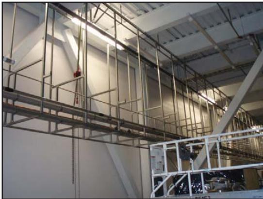
*Piping system vulnerable to "out-of-phase" movement*
