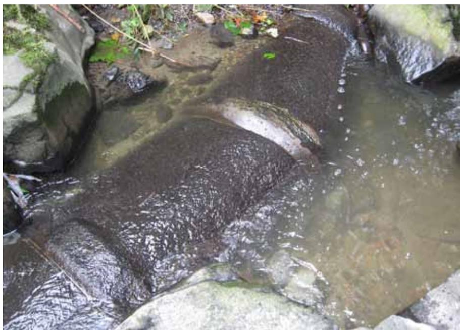
**District staff discovered that sewer lines and several manholes, which previously were buried beneath the stream, had been exposed.** PACE Engineers/SWSSD
