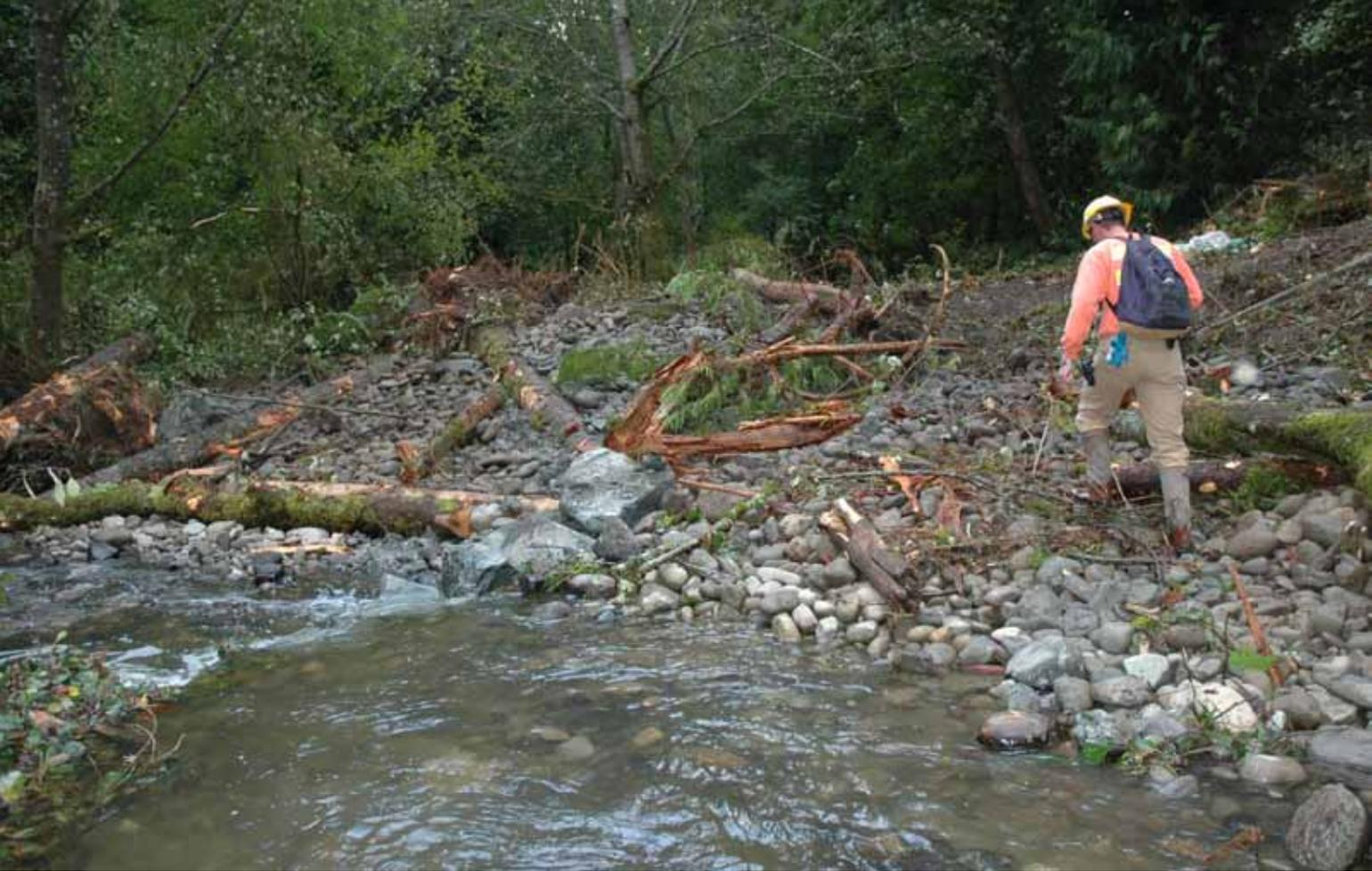
**Post-construction, the stream channel has been raised to its 1966 conditions and constructed to minimize future erosion.** PACE Engineers/SWSSD
